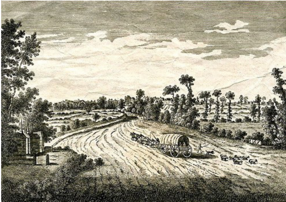
A 19 th Century Turnpike Road.
